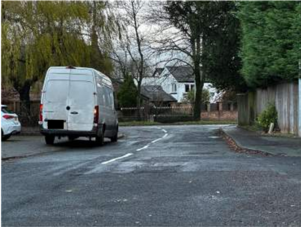
Stockton Road / Knutsford Road Junction
